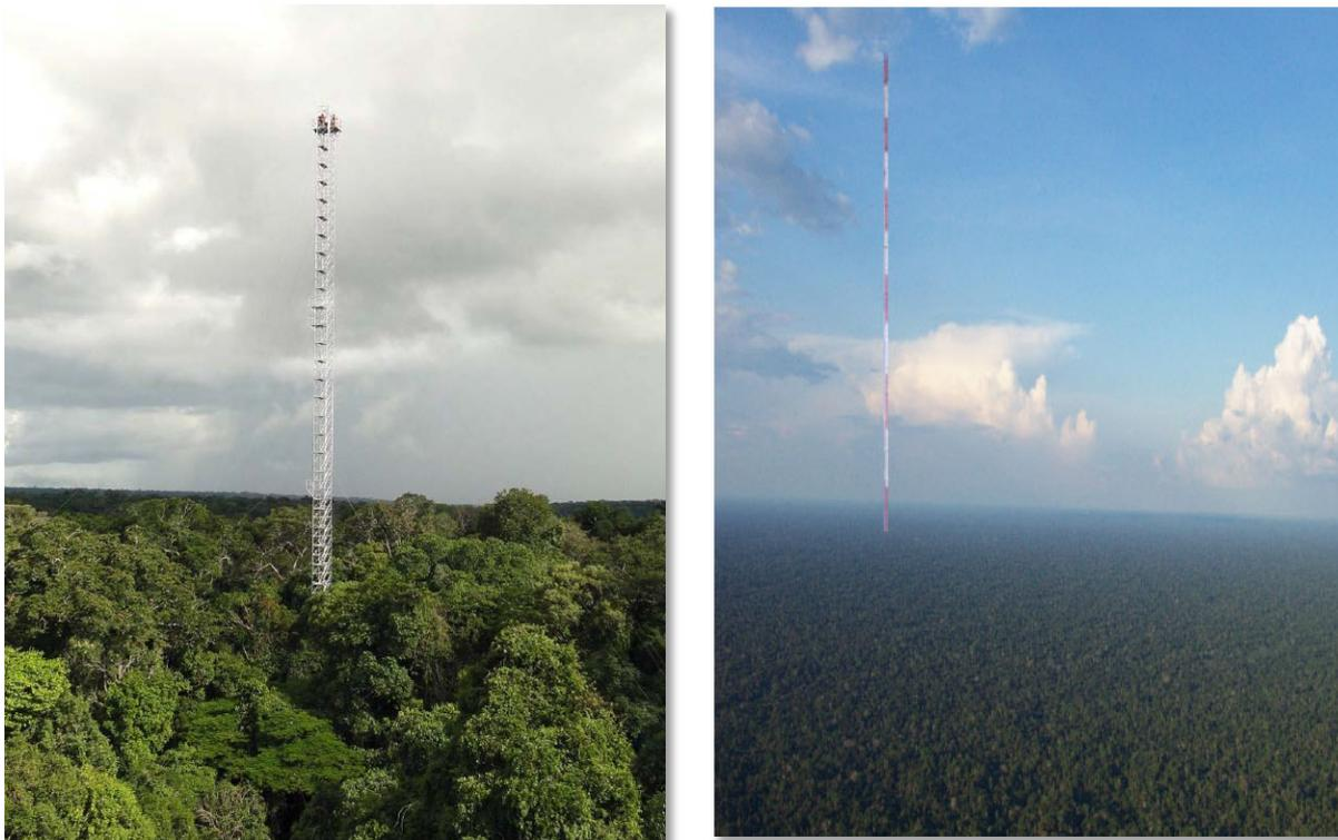
**Figure 7** - ATTO site: Picture of the 85 meters tall tower at the left that is being used for aerosol and trace measurements and the proposed 320 tall tower (right) under construction.
